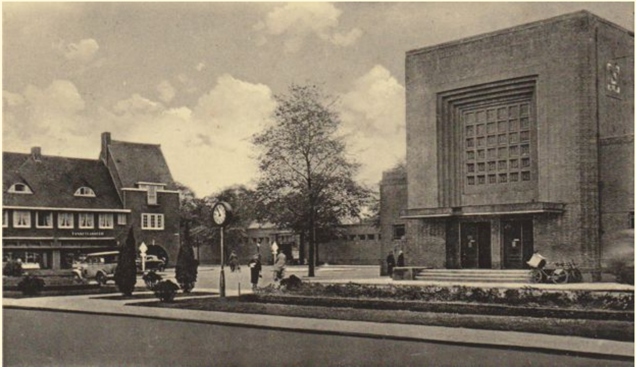
Station Naarden-Bussum in 1934, architect H. Schelling
